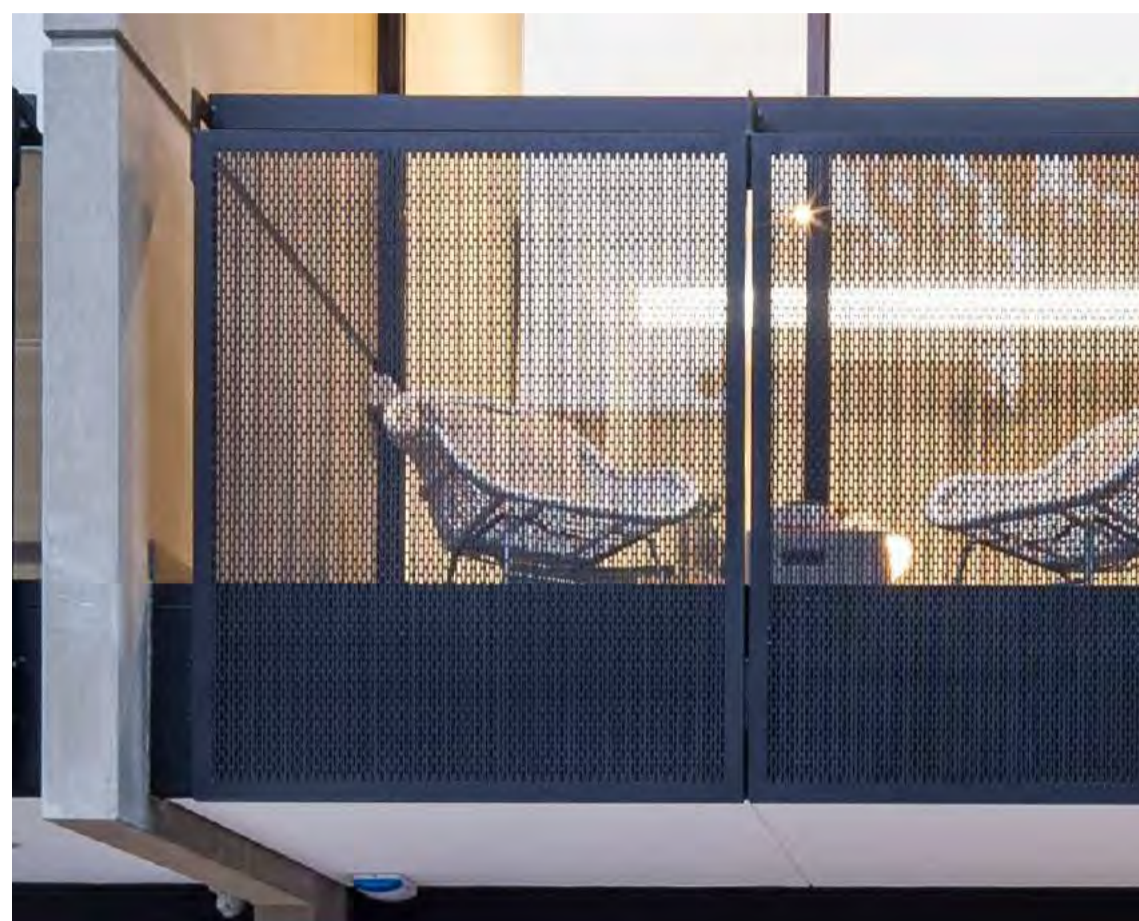
PERFORATED STEEL MESH BALUSTRADE
